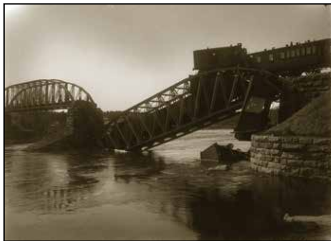
Sabotaged railway bridge
